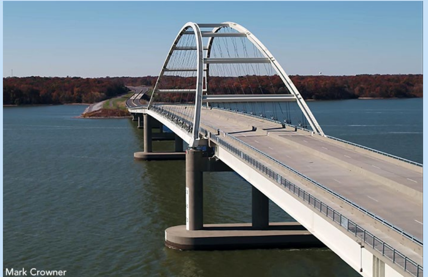
Eggner Ferry Bridge (Over Kentucky Lake near Paducah, KY)
