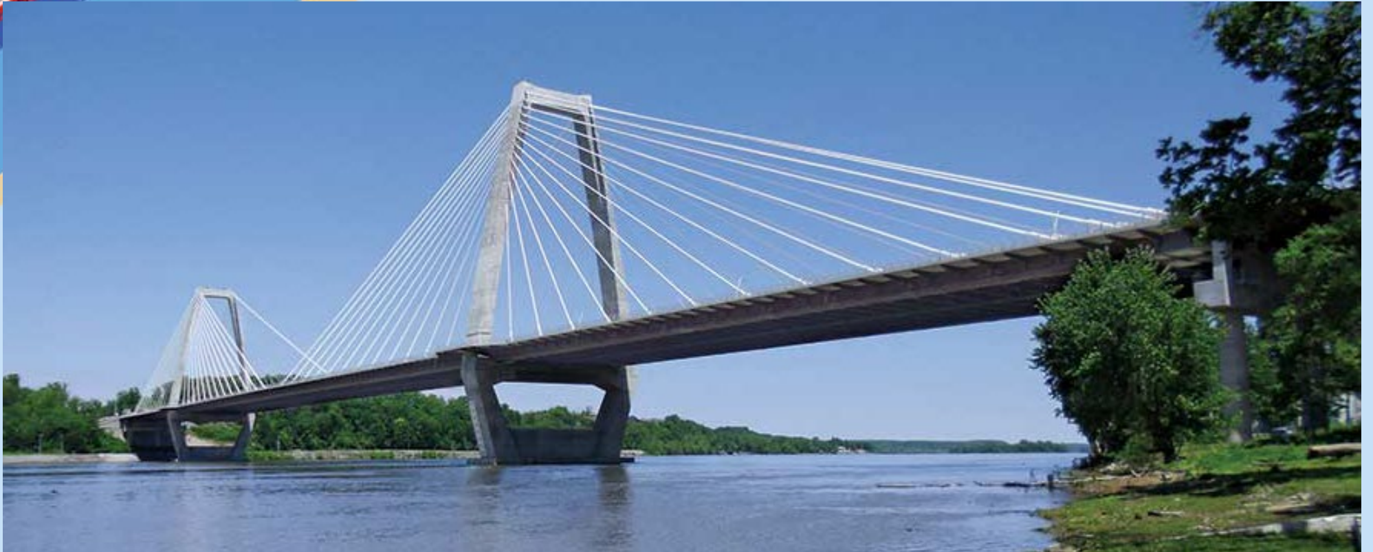
Lewis and Clark Bridge (Louisville, KY)
