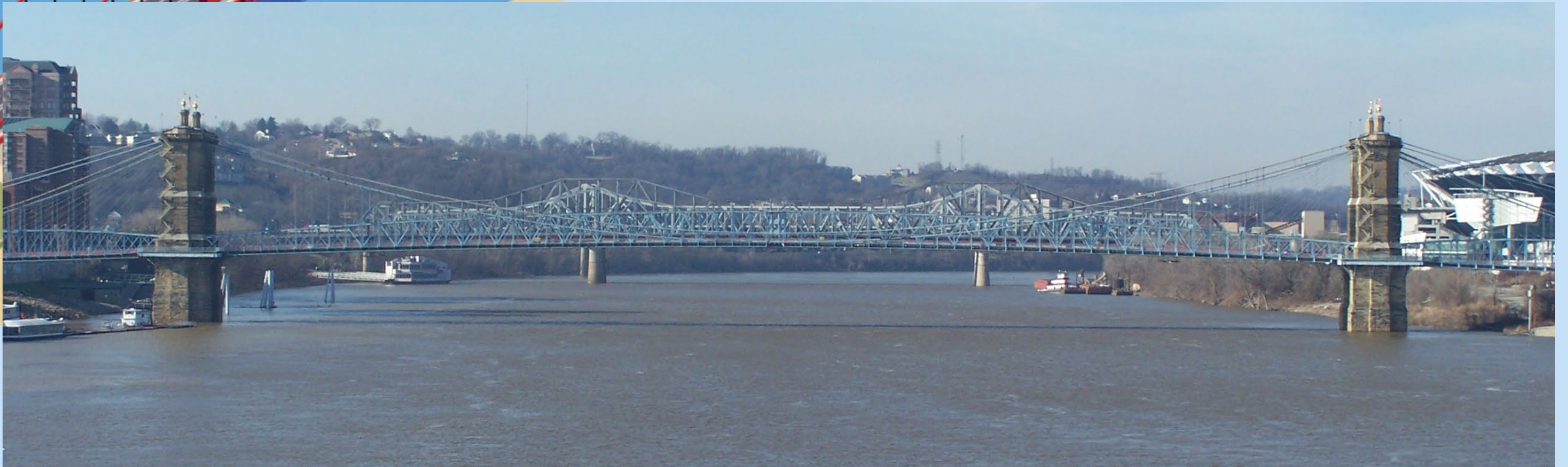
Roebling Suspension Bridge
