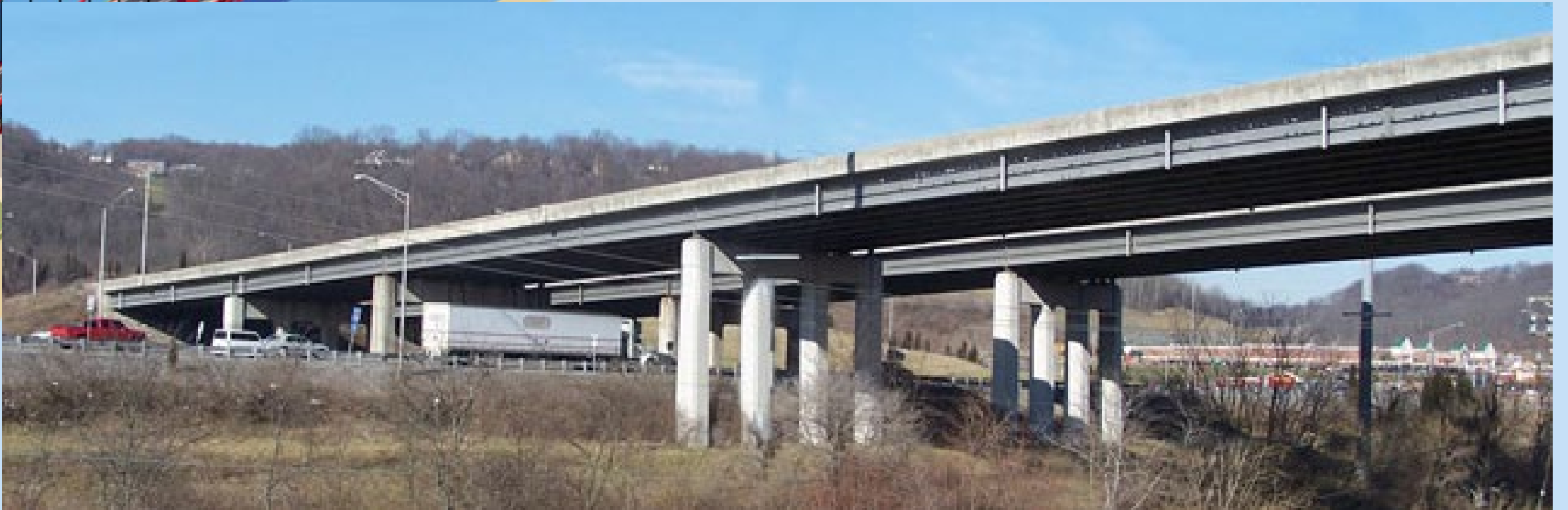
A Standard Beam and Girder Bridge in Northern Kentucky
