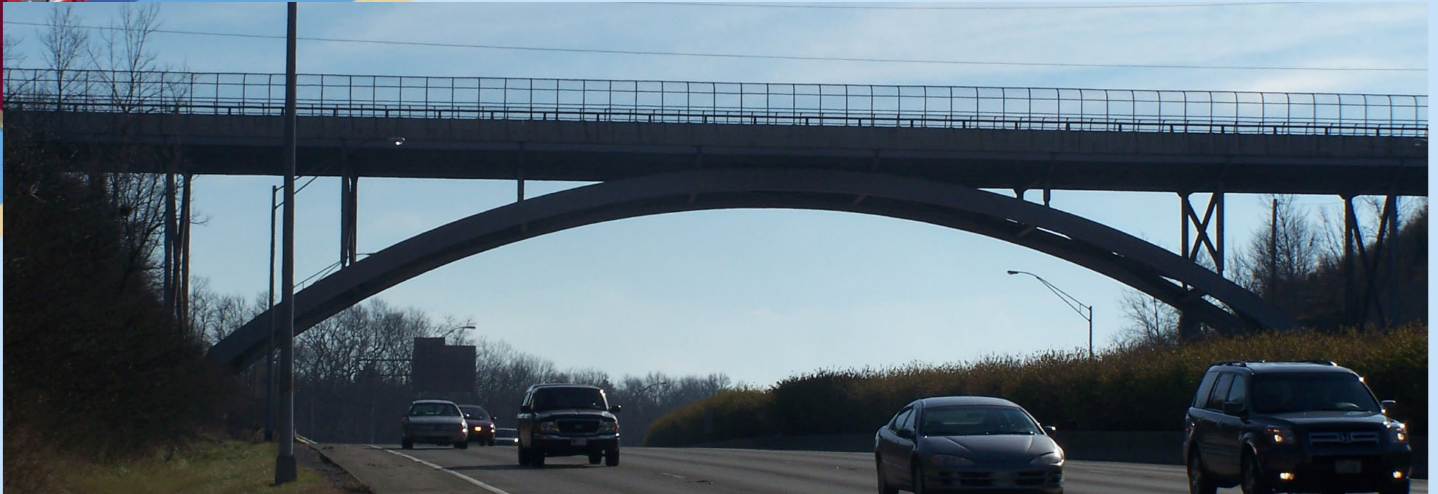
Deck Arch Bridge in Northern Kentucky near Cincinnati
